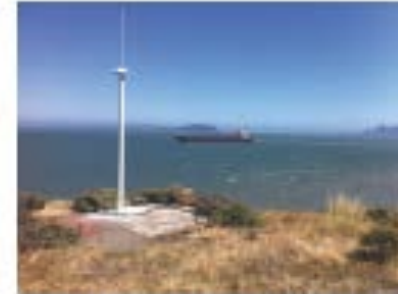
Figure 2. IOOS operates the nation's only network of land-based high-frequency radars (pictured above) that provide continuous, real-time mapping of the speed and direction of surface currents in coastal waters.
