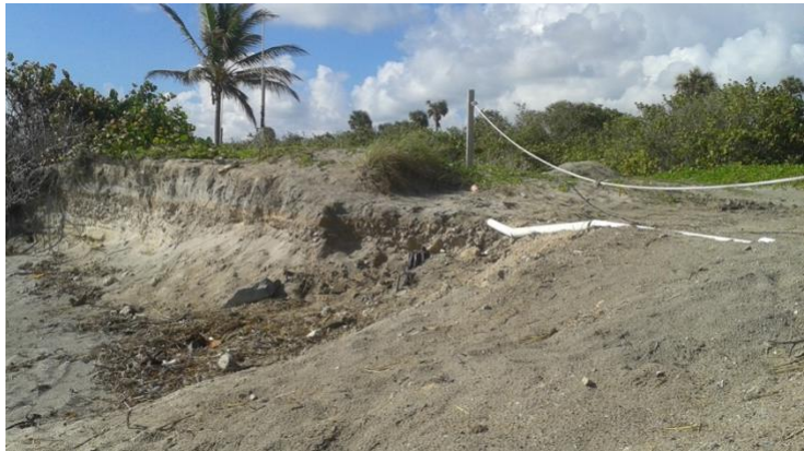
Figure 3. Hurricane Irma damage (2017) to HFR off the coast of Miami, FL. Overwash from the hurricane exposed and damaged the cables, resulting in total loss of communications. Image credit: UM RSMAS
