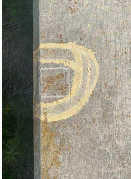
*Image 3 (left): North Carolina DOT benchmark with RTK/RTN placed vertically above the BM. Note the DOT metal disc has yellow paint around it to help identify it more easily.*
