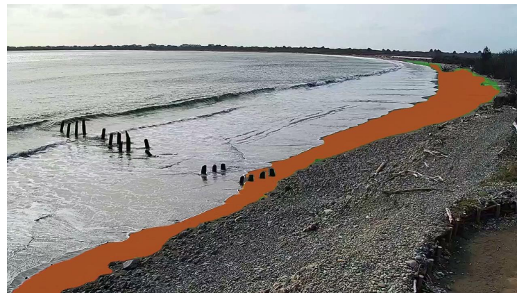
Sand Tracking (Ocean Shores west)
